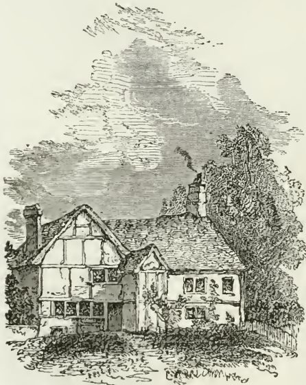
Milton's Cottage at Chalfont.
